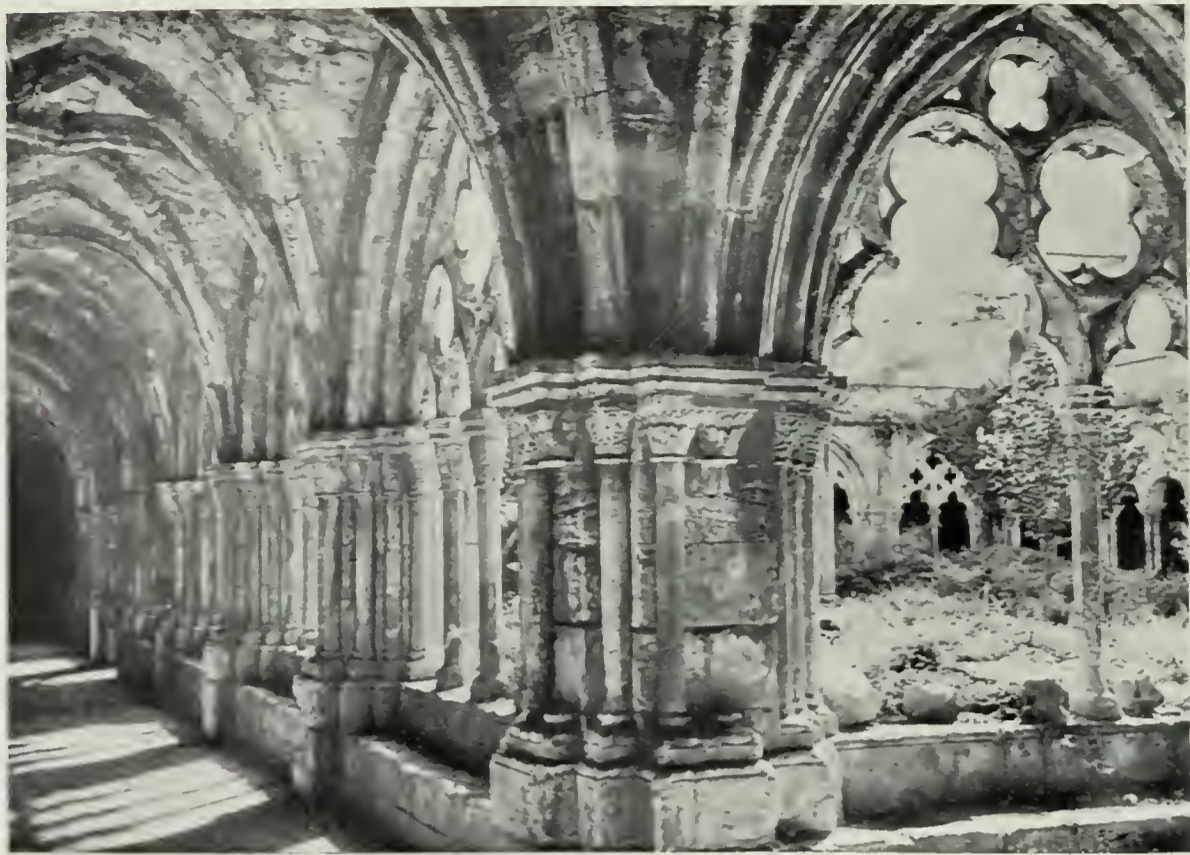
INTERIOR VIEW OF THE CLOISTERS, POBLET (PROVINCE OF TARRAGONA)
